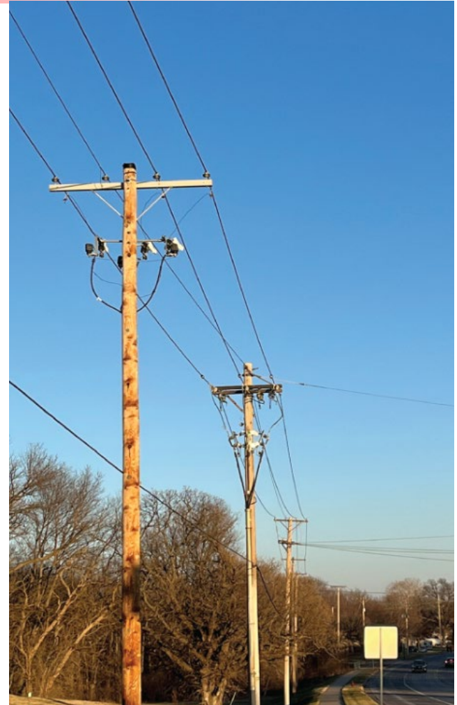
Figure 1.5 A 12.47-kV primary feeder. 21
