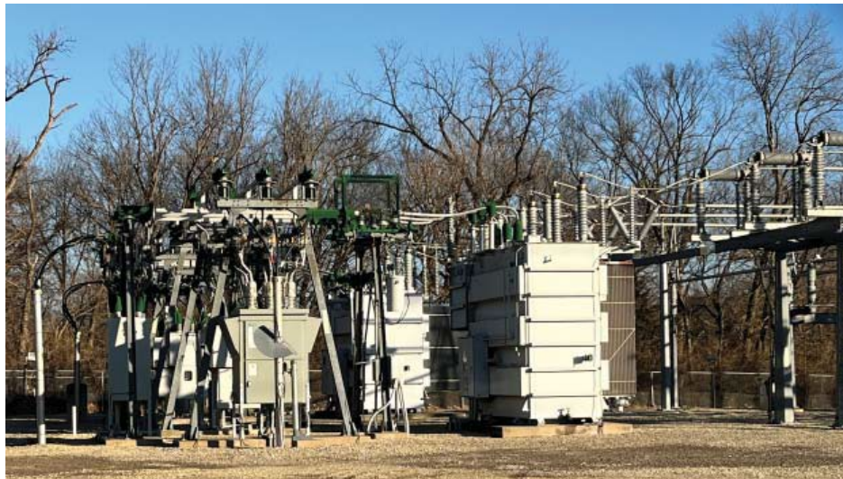
Figure 1.3 The 12.47-kV side of the substation showing the transformer, circuit breakers, and the rest of the equipment.
