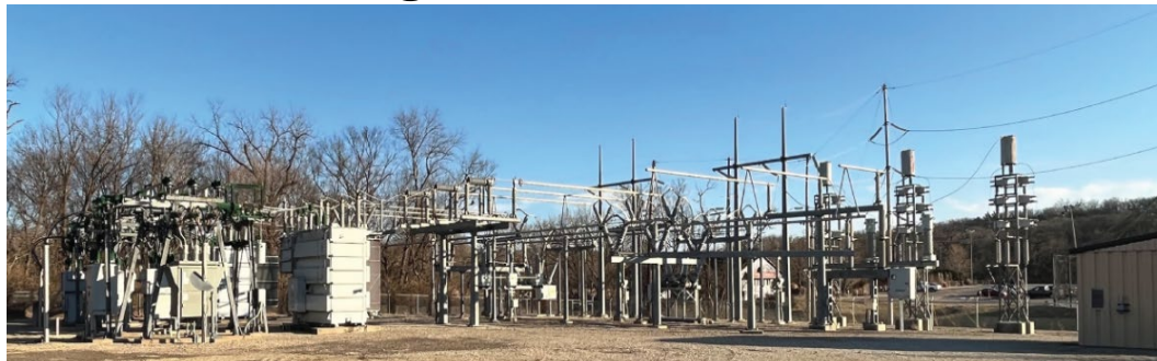
Figure 1.2 A 115-kV to 12.47-kV step-down distribution substation.
